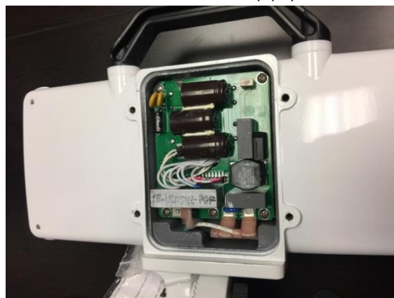
Internal Power Supply
